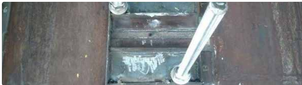
3. Finished application (exterior)
