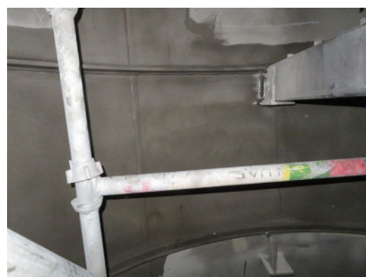
HVTS cladding applied on internal shell
