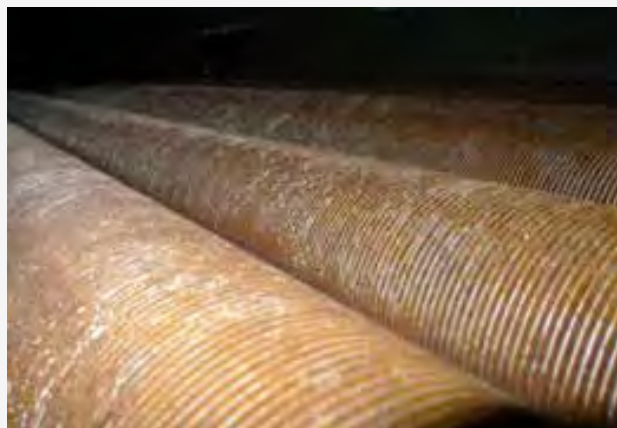
Figures 6&7. Before and After Fouling Removal Pictures. Part 1.
