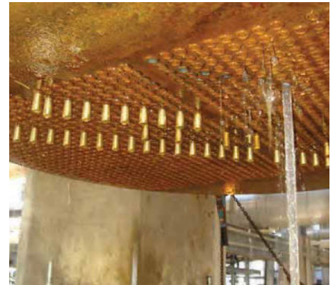
Tubes Running Clear After Enhanced Tube Tech Cleaning
