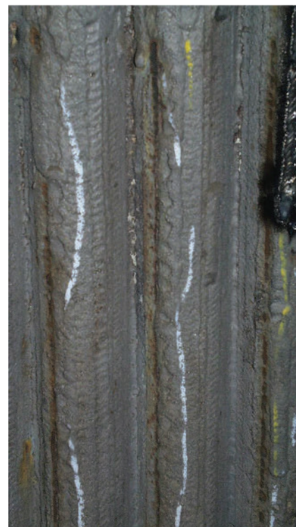
Field services – on site weld overlay
