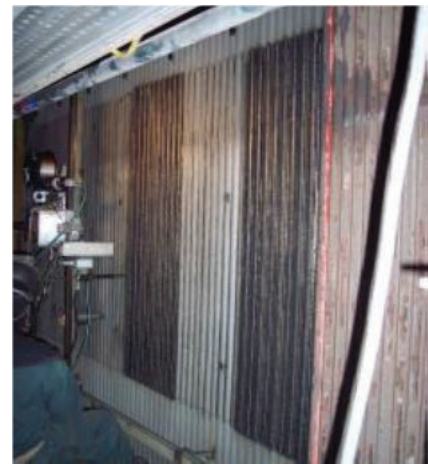
Field services – on site weld overlay
